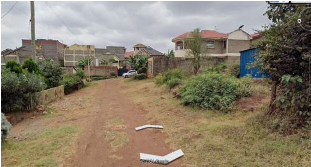
Photo: 11. This Michuki service road would benefit from trimmed vetiver hedgerows on either side
