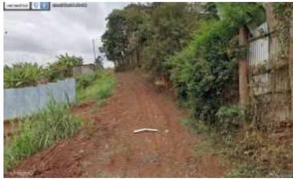
Photo: 16. Another poorly maintained road that takes discharge of effluent from adjacent properties
