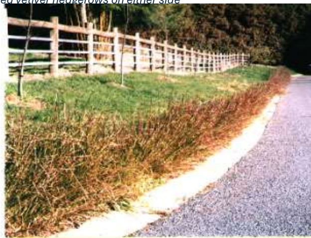
Photo: 19. This roadside vetiver prevents sediment from entering the drain, reducing road maintenance costs.
