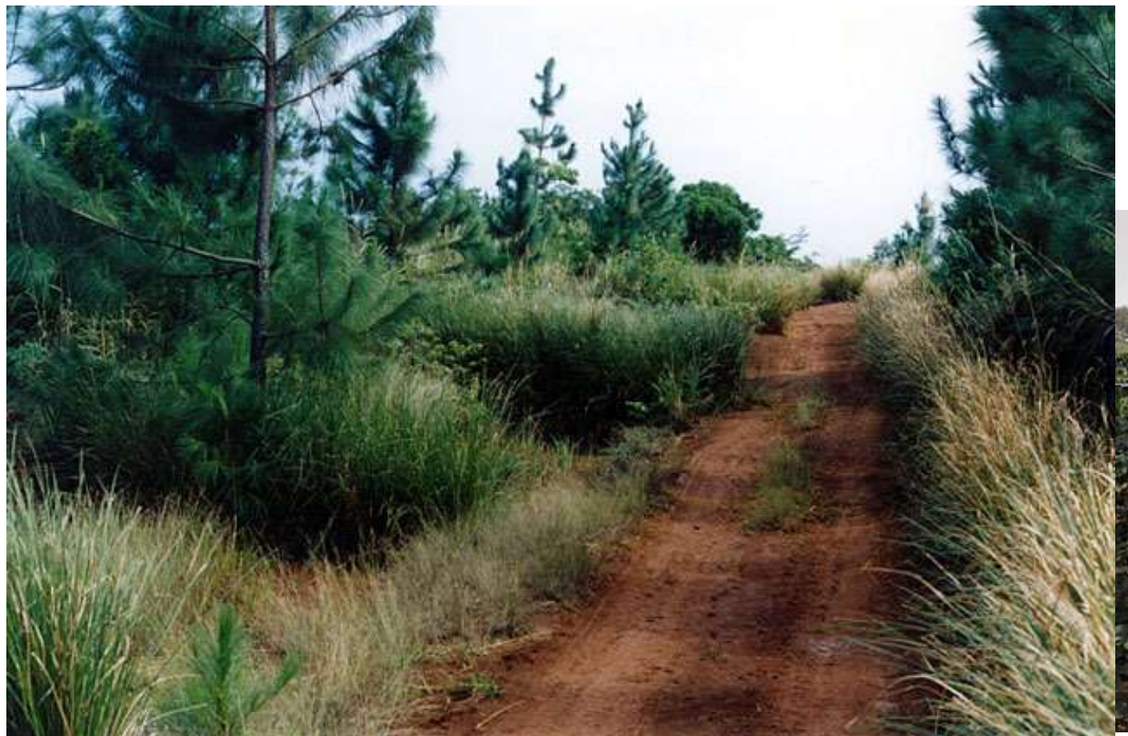
Photo: 3 Vanuatu (South Pacific - Vetiver planted on road shoulder and vetiver miter drains that discharge rainwater from road to adjacent land
