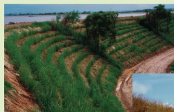
Farm dam stabilization and protection
