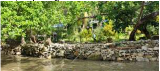
Mangroves, stonewall and Vetiver for coastal erosion (new planting)
