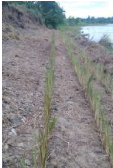
Demonstrating to PE team on the planting method for riverbank protection works
