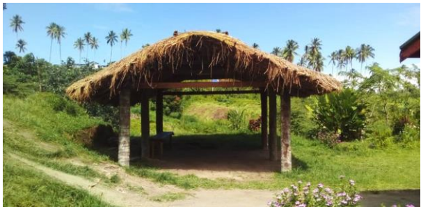
Roof thatching in Kokopo, East New Britain Province
