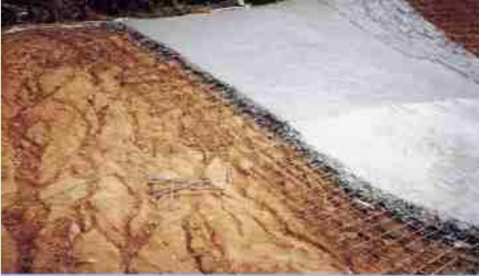
3-5 混凝土挡墙有时也会崩塌 Concrete wall destroyed if slope was not fixed
