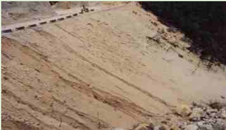
3-1 新修公路很易遭受土壤侵蚀 New highway subject to erosion
