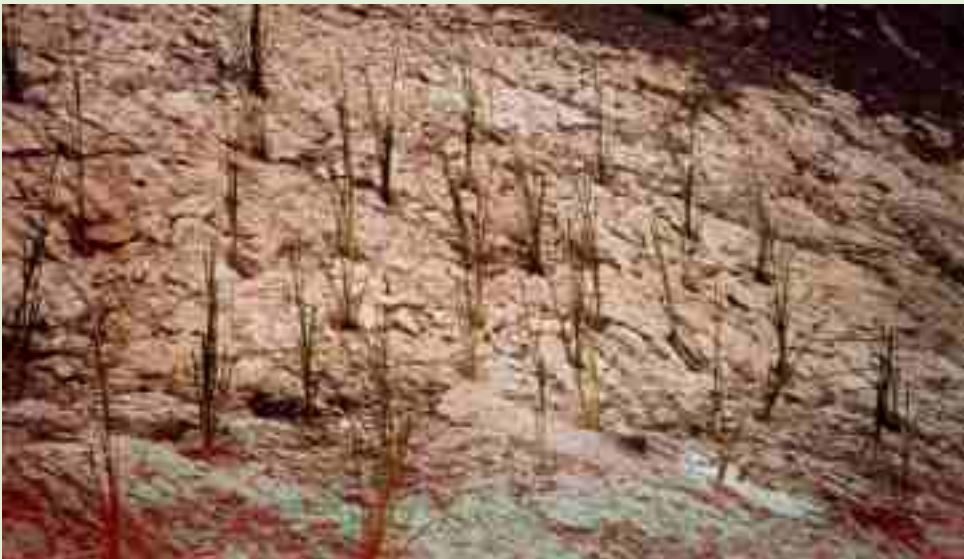
5-7 在岩石上打洞种植香根草 Drill holes and planted vetiver on the rock
