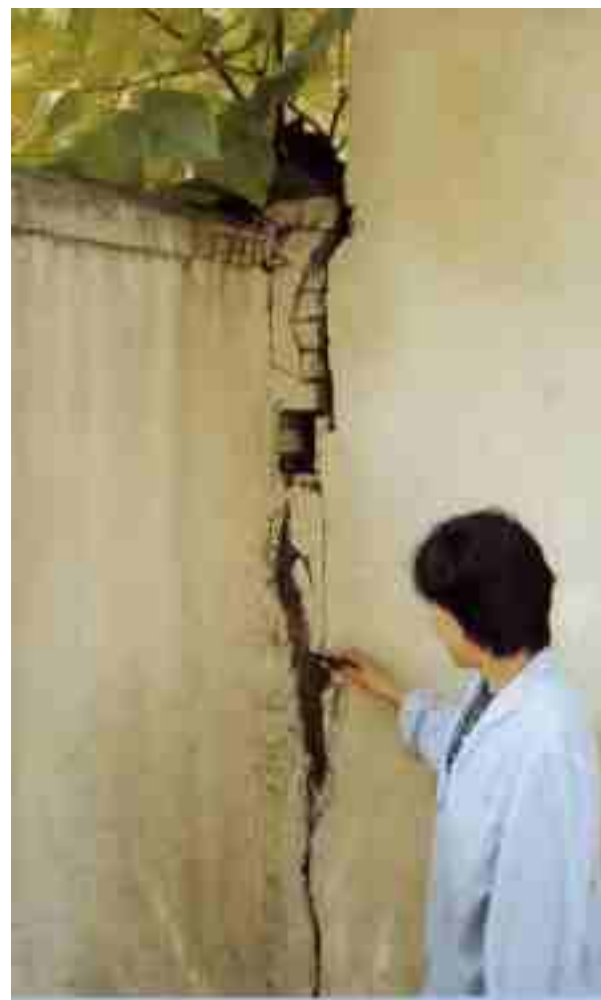
1-4 某些树木根系有时可挤裂建筑物 Some roots may split construction
