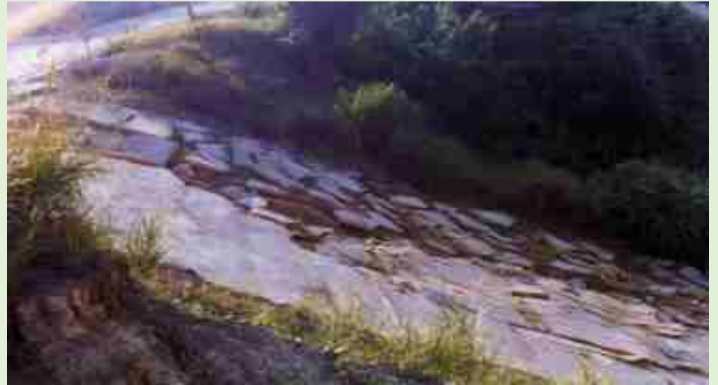
3-6 石砌挡墙因侵蚀而破坏 The rock wall destroyed by erosion
