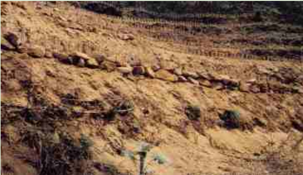
2-5 用小石块护坡再栽上香根草 Protect slope by small stones and then plant vetiver
