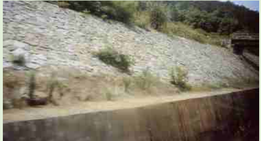
3-2 混凝土常用于保护道路边坡 Concrete usually for road embankment protection
