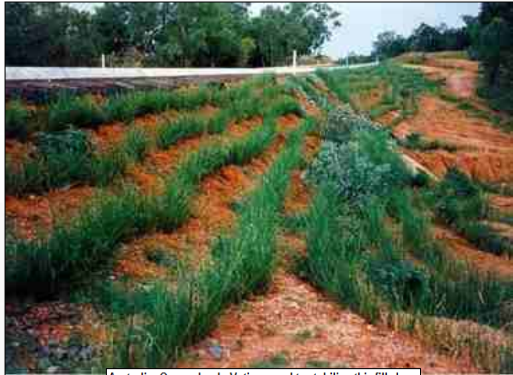
Australia, Queensland - Vetiver used to stabilize this fill slope
