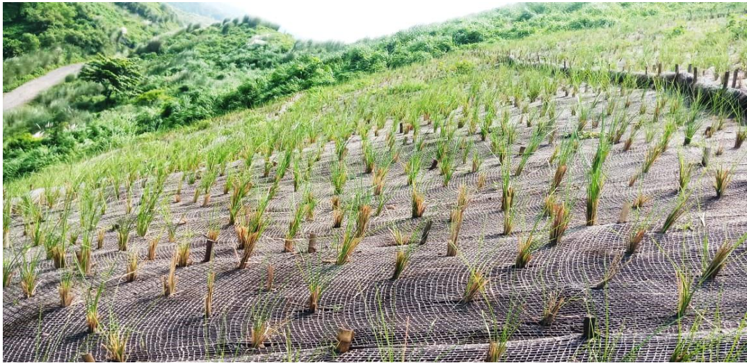
Vetiver plant growth on bioengineered fly ash mount
