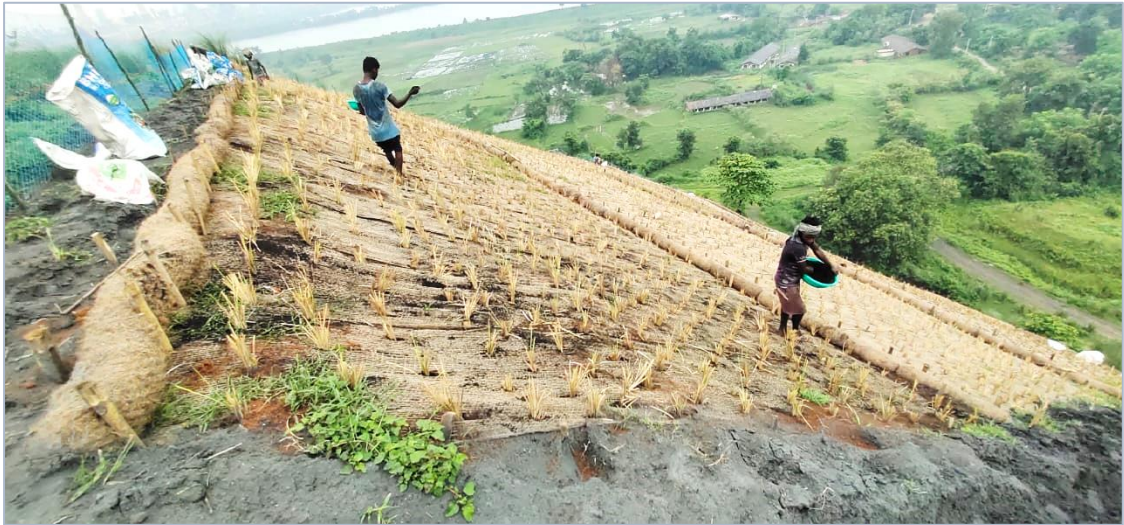
Plantation on compacted Jute geotextiles mulched area
