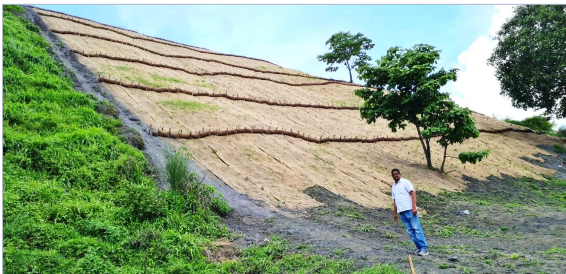
Fixing of Jute geotextiles & Coir logs for ash sliding control and compaction of site for plantation
