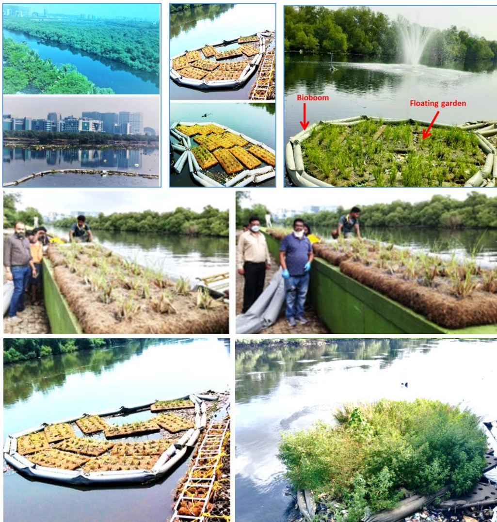
Mithi River Treatment system for Sewage. Effluent, Saline and Tidal Impacted area by In-situ Bio-phyto remediation
