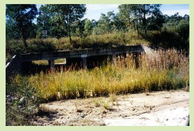
Australia, Queensland. Railroad tunnel entrance, drain underpass and railway batter cut all stabilized with vetiver grass hedgerows at 1/20 of the cost of standard practices.
