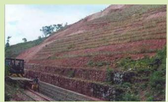
This 200 km railway in eastern Madgascar was devastated by cyclones due to lack of maintenance and cultivation in the right of way. A plan linking the railway, farmers and vetiver was put in place, with a result that the railroad is now stable, operates without slope failure, and the farmers have better incomes
