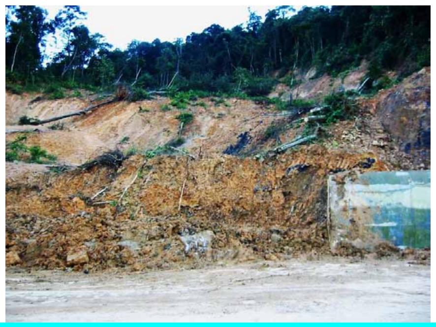
02/2003. Large landslide in weak, clay rich, highly saturated soil at Da Deo Pass, one of the most problematic, about 1km long, section.
