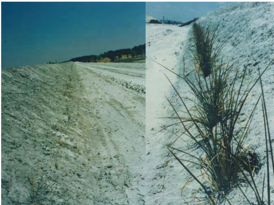
**Figure 49.** Gold mine tailings dam before (left) and after three month of Vetiver planting (right) (Tony Tantum pers.com.).
