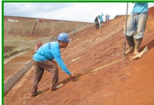
LEAD MAN MEASURING THE SURFACE RUN OF THE SLOPE
