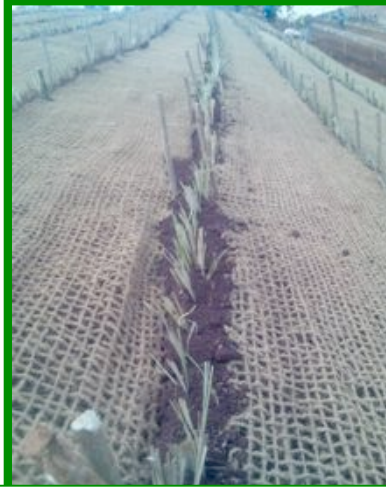
BACKFILLED VETIVER ROWS
