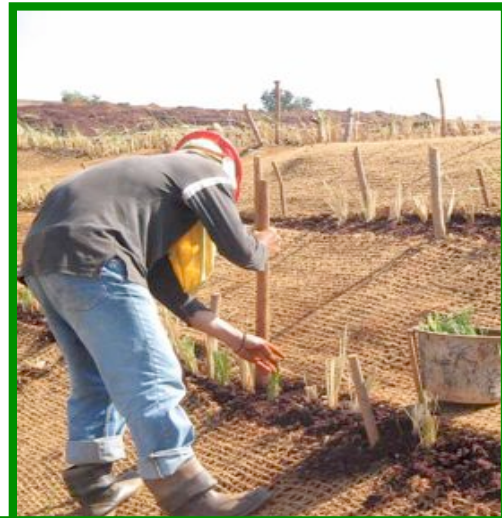
REPLACEMENT OF DEAD PLANTS
