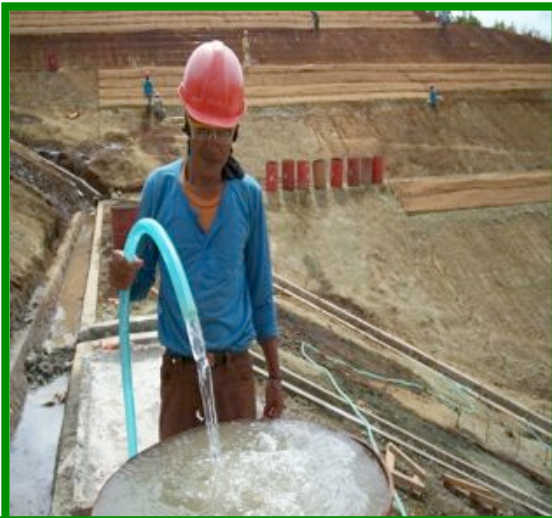
WATER IS COLLECTED IN CONTAINERS FOR USE ON THE VETIVER GRASS
