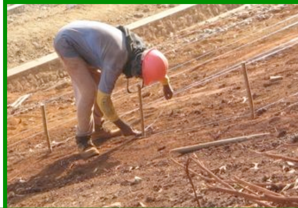
NYLON LINES ARE STRETCHED AND STAKED ON THE GROUND WITH KAKAWATE CUTTINGS
