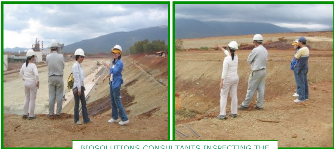
BIOSOLUTIONS CONSULTANTS INSPECTING THE SITE WITH ENGR HAMLIG
