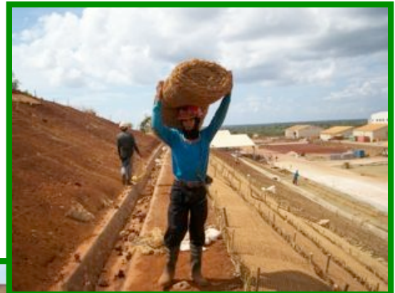
BACKFILLED VETIVER ROWS
