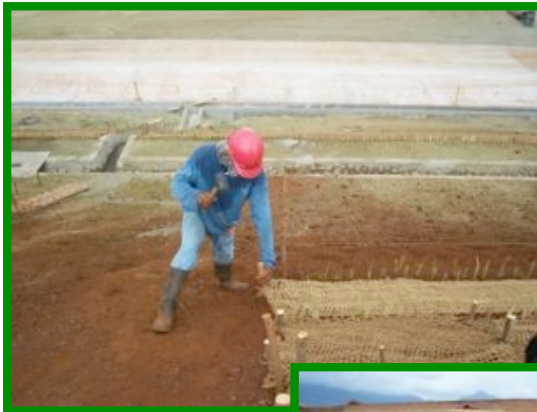
BACKFILLED VETIVER ROWS
