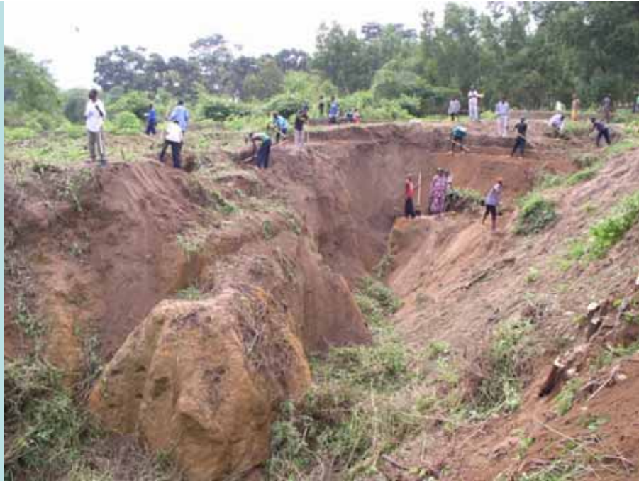
Terracing the ravine walls at Kikwit
