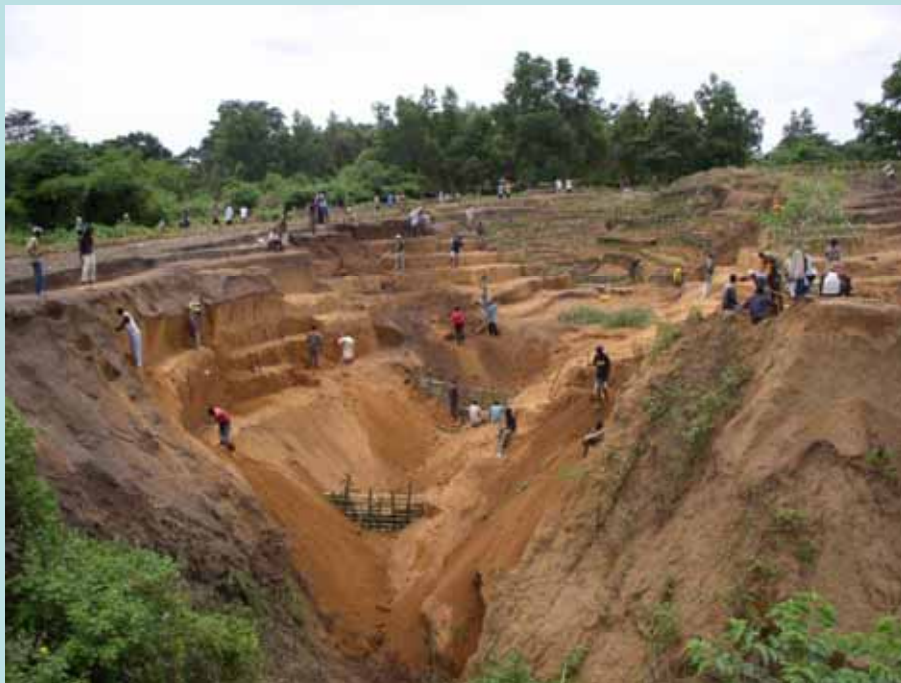
Terracing the ravine walls at Kikwit
