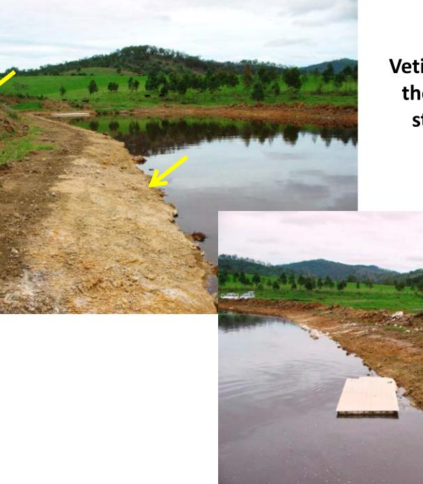
Vetiver planting on the banks of the storage ponds Two months after planting on banks of the storage ponds, irrigated with pond effluent
