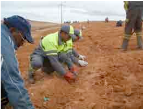
Preparing furrows for contour planting, solid Disposal site (Oujda)
