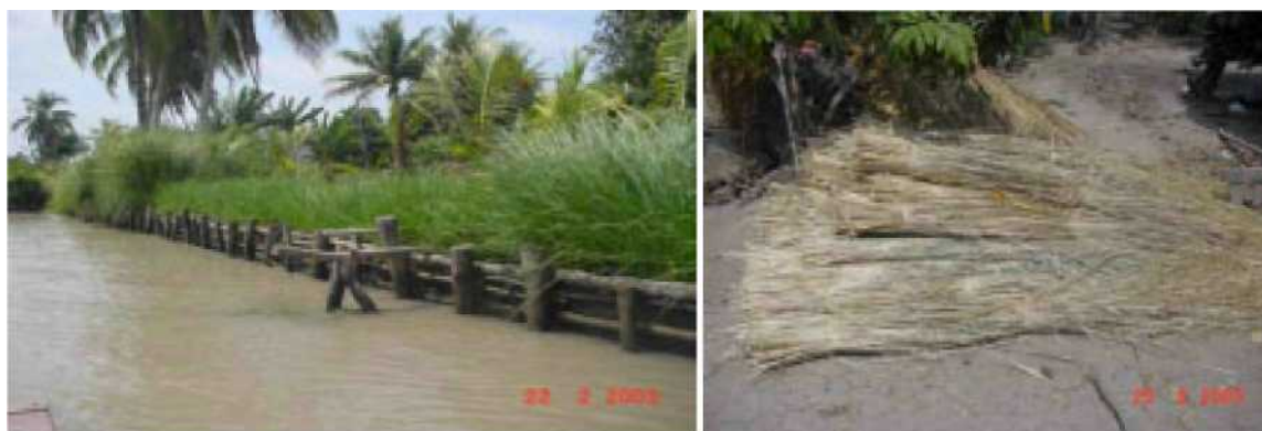
Photo 7. Reinforcing the wooden structure (Left) and being prepared for string
