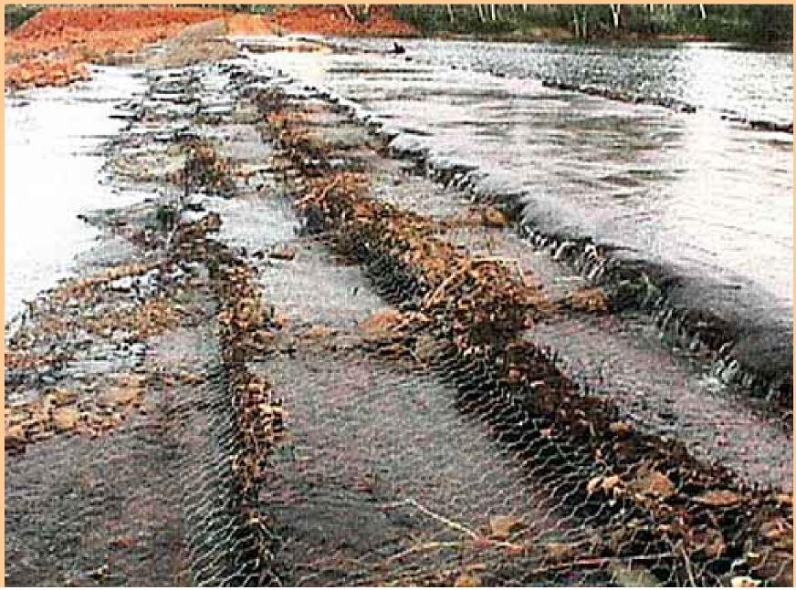
This causeway was again flooded 8 months after planting with flow up to 3m deep. Despite the young age vetiver plants were sufficient to withstand the high velocity flow and stop the erosion.
