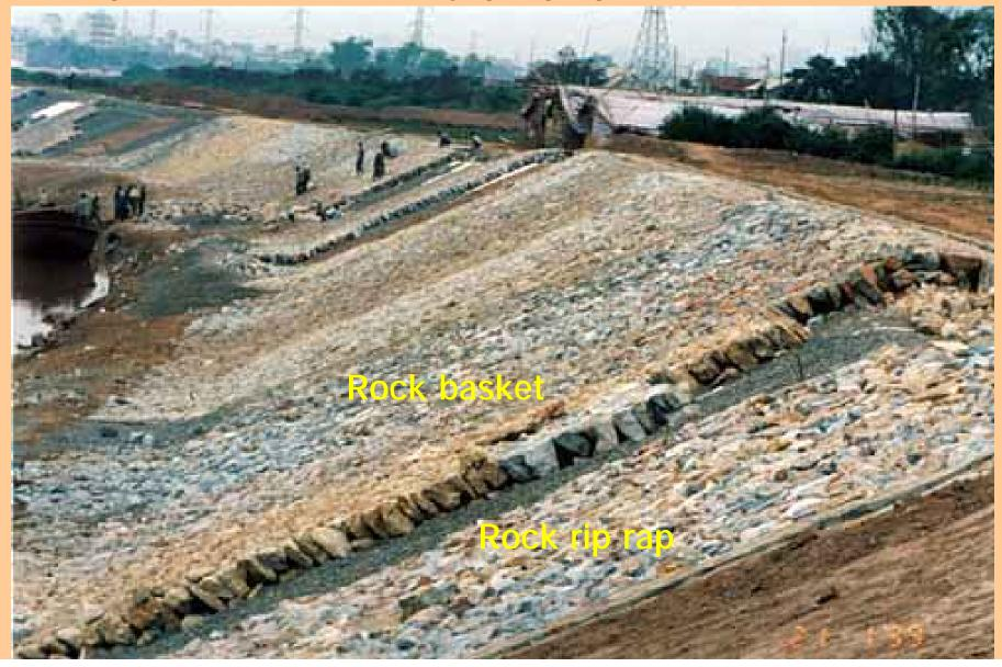
But this method provided no protection as this bank had been previously covered by similar rock baskets. Remnants of the old rocks which collapsed in the last flood, were still visible in the river.
