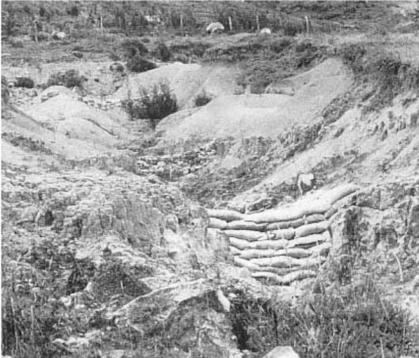
A common practice, recommended by authorities throughout the world, is the gully check. This is typically a "dam" of masonry, rocks, sandbags, logs, or brushwood. Thousands are installed in isolated catchments in every country.
