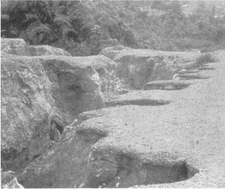
Roads commonly spawn severe erosion. The smooth, flat surface collects water and cascades it over the banks, washing out the slopes below. Slopes above the road are also erosion prone, especially as they are often extremely steep. Embankments freshly cut out of hillsides or built up from fill are particularly vulnerable. The damage can be immense—to the roads, to the neighbors, and to the environment in general.
