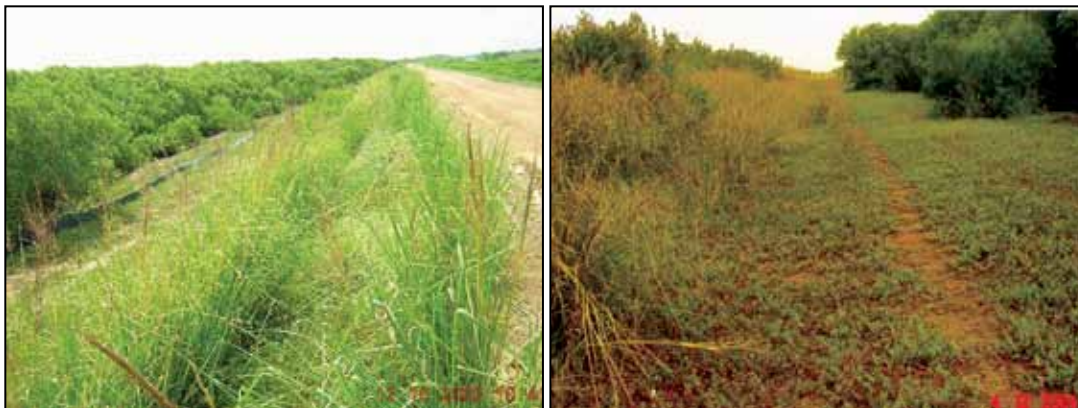
Photo 17: Planted behind natural mangrove on an acid sulphate soil sea dike in Go Cong province, vetiver reduces surface erosion and fosters the re-establishment of local grasses.
