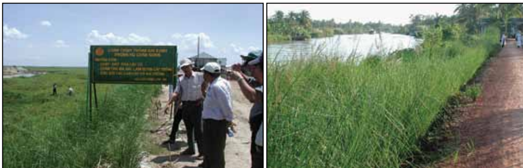
Photo 15: In An Giang vetiver stabilizes a river dike (left), and a natural river bank (right).
