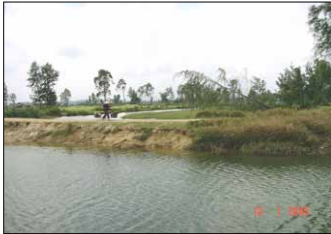
Photo 23: The right section of this rural road in Quang Ngai is protected by vetiver; the left section is unprotected.
