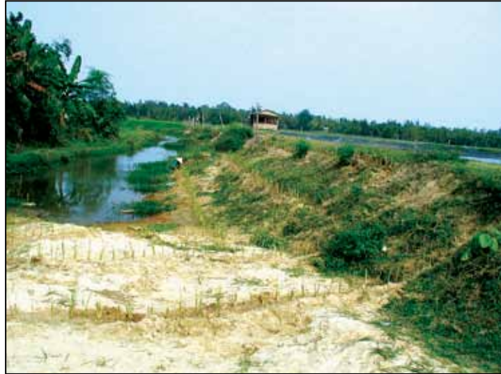
Photo 21: Vetiver protects a shrimp pond near a natural gully that drains water into a river (Da Nang province); this model was established as part of the first vetiver project financed by the Royal Netherlands Embassy in Vietnam.
