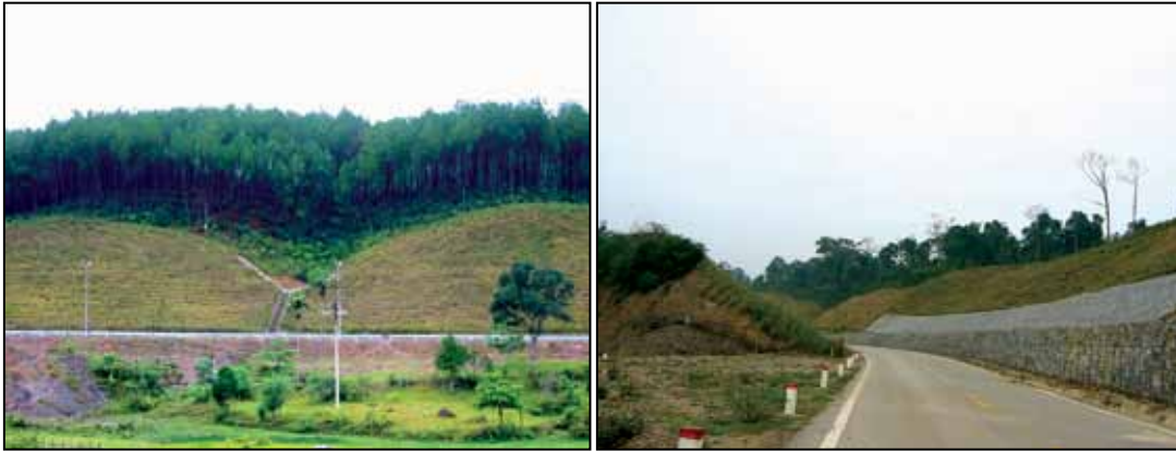
Photo 19: Left: Vetiver stabilizes cut slopes along the Ho Chi Minh Highway; right: both alone and in combination with traditional measures.
