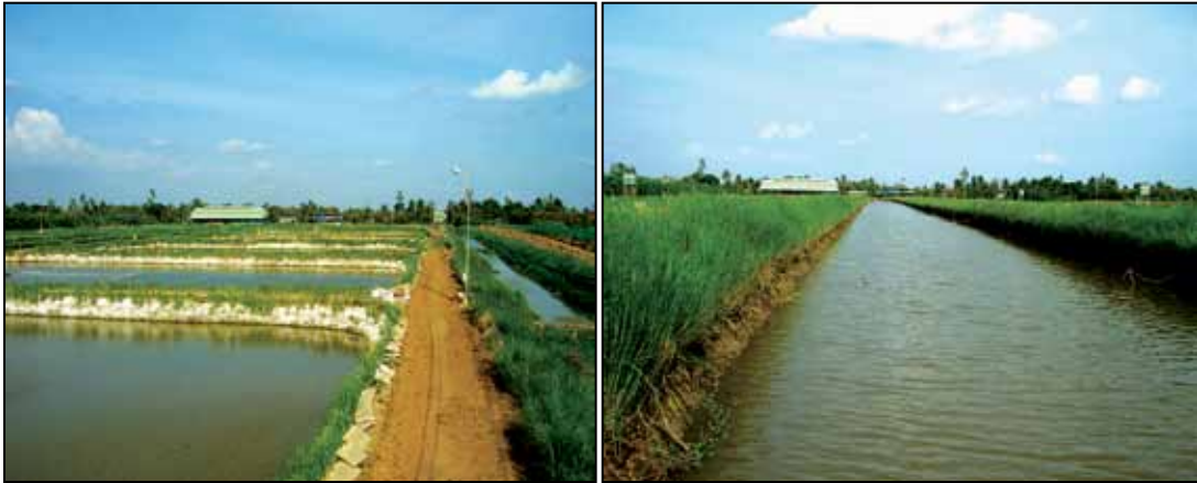
Photo 3: Erosion control and wastewater treatment at a freshwater fish farm in the Mekong Delta.
