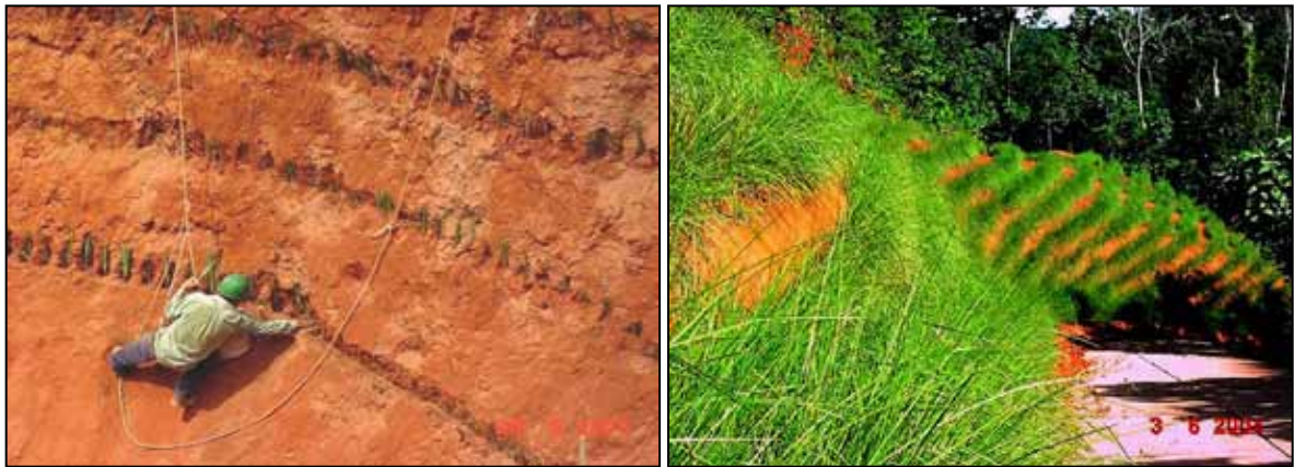
Photo 10: Left, Bauxite mine at Los Pijiguaos, Venezuela protected with vetiver (note the planting of the steep slope by using ropes).
