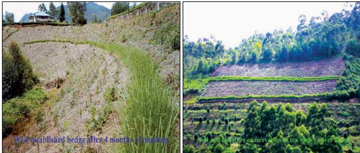
Photo 3: Vetiver planted on very steep slopes at about 1,700 m a.s.l. In the Munnar area of the Western Ghats of India in the state of Kerala. This major tea growing area suffers from serious erosion. All the estates in the area are now adopting the Vetiver System.
