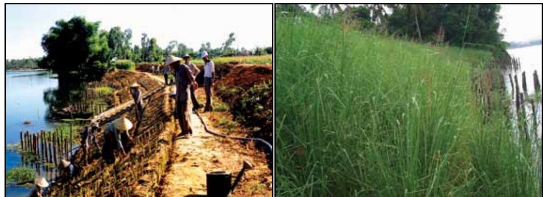
Photo 14: Left: Community members plant vetiver; right: November 2005: bank remains intact following the flood season.
