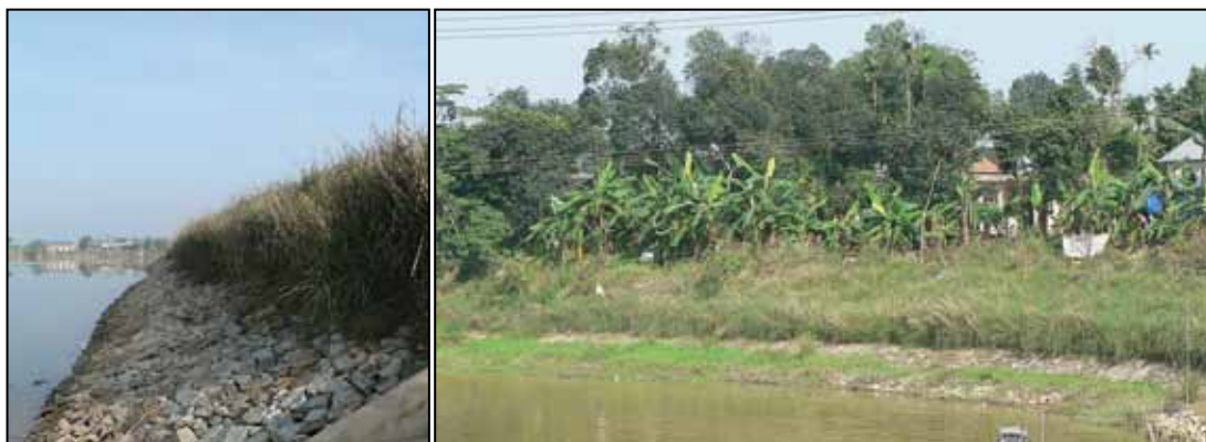
Photo 10: Left: Vetiver and rock riprap (upper) and concrete frame (lower) protect an embankment; right: a bend on Perfume Riverbank in Hue.
