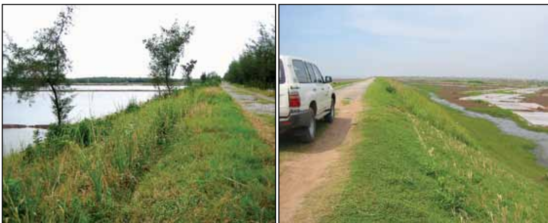
Photo 18: In North Vietnam; left: Vetiver planted on outer side of a newly built sea dike in Nam Dinh province; right: on the inner side of the dike, planted by the local Dike Department.
