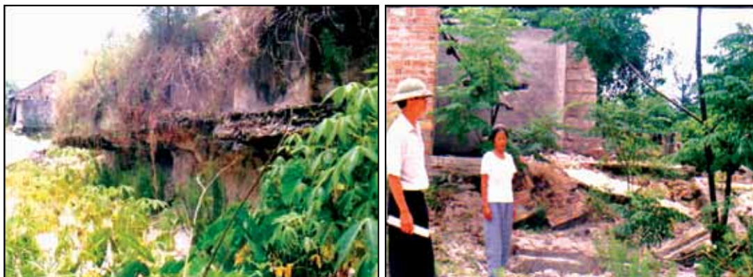
Photo 2: Sand flow in Le Thuy (Quang Binh) in 1999: the foundation of a pumping station (left) and the foundation of this woman’s three-room house is being undercut by moving sand (right).
