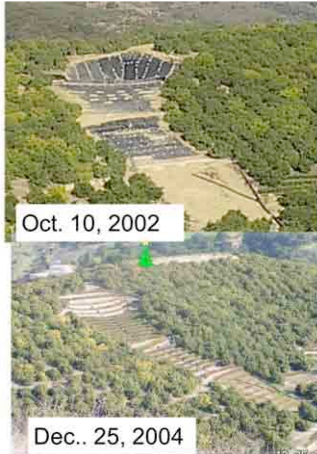
Protection of mudslide area in southern California using vetiver grass – photo by Jerry Coyle
