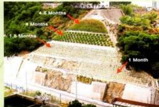
4-5 Months 3 Months 1.5 Months 1 Month CED Contract No. GE/2000/04 Landslip Preventive Works for Slopes and Retaining Walls in Tsuen Wan and Kwai Tsing Districts Feature No. 75W-C/C47 at Kwai Shing Circuit
