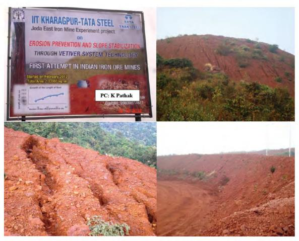
**Figure 76.** The old waste dump is highly erodible and steep (top and bottom left), and re-shaped to 40 (bottom right).
