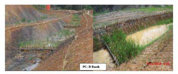
**Figure 59**. Vetiver planted for channel bank stabilization (along the channel) and sediment traps (cross the channel). Source: www.vetiver.org
