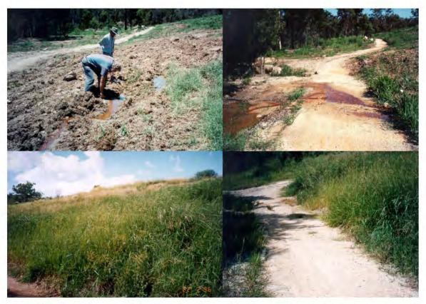
**Figure 40**. Leachate after rain on the side slope of the old landfill mound (top), within a year Vetiver completely stopped the leachate seepage (bottom).
