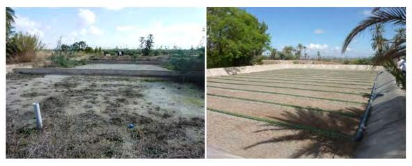
Figure 22. The dysfunctional wetland using Typha (left) and seedbed ready for Vetiver planting (right).
