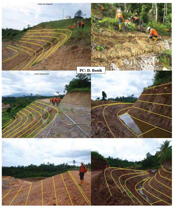
**Figure 48**. Design and application of Vetiver grass technology throughout extensive infrastructure and drainage. Source: www.vetiver.org.
