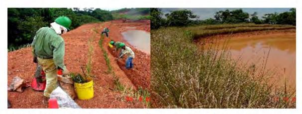
**Figure 65.** Vetiver planted for reinforcement of lagoon dikes (left) and 14 months after planting (right). Source: Luque et al., 2006.
