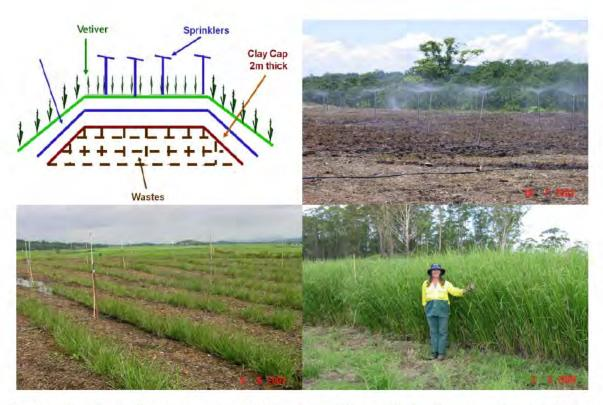
**Figure 35**. The Vetiver treatment at Stott Creek landfill mound: the diagrammatic cross section of the mound (top left), Vetiver irrigated every day with leachate after planting (top right), two (bottom left) and twelve (bottom right) months after planting.
