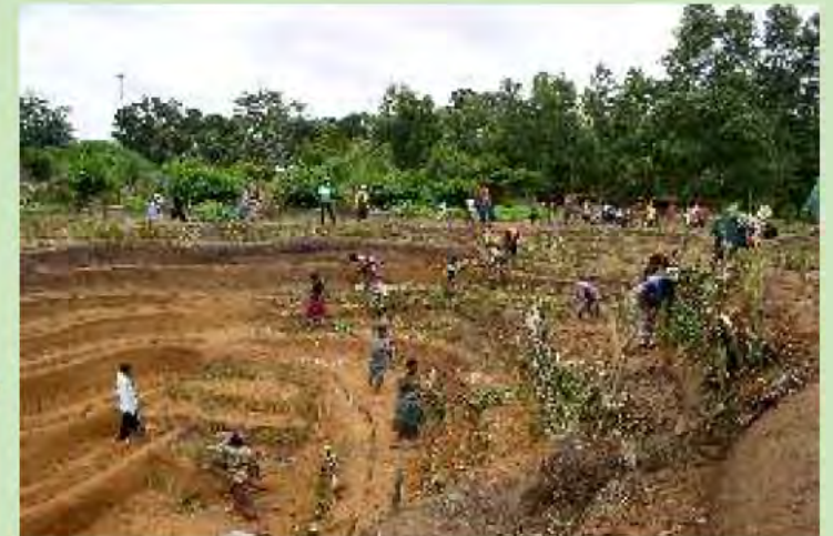
Congo (DRC) - A reshaped urban gully being stabilized with vetiver grass
