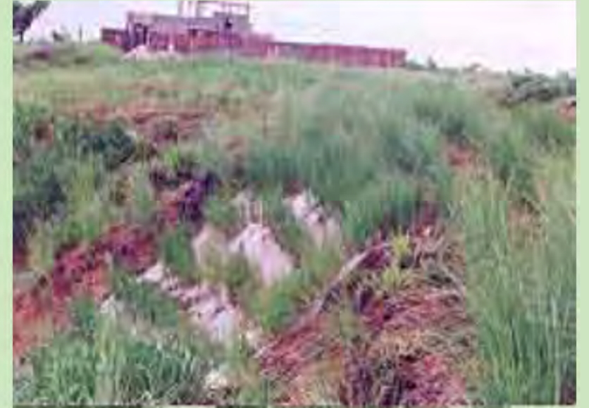
Mexico - Oaxaca. Stabilizing a cliff with vetiver
