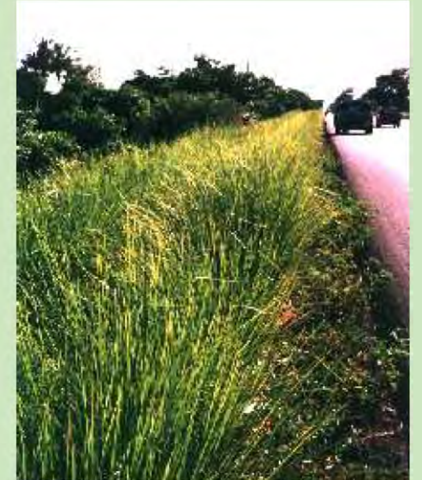
El Salvador - mature vetiver hedge protecting road embankment
