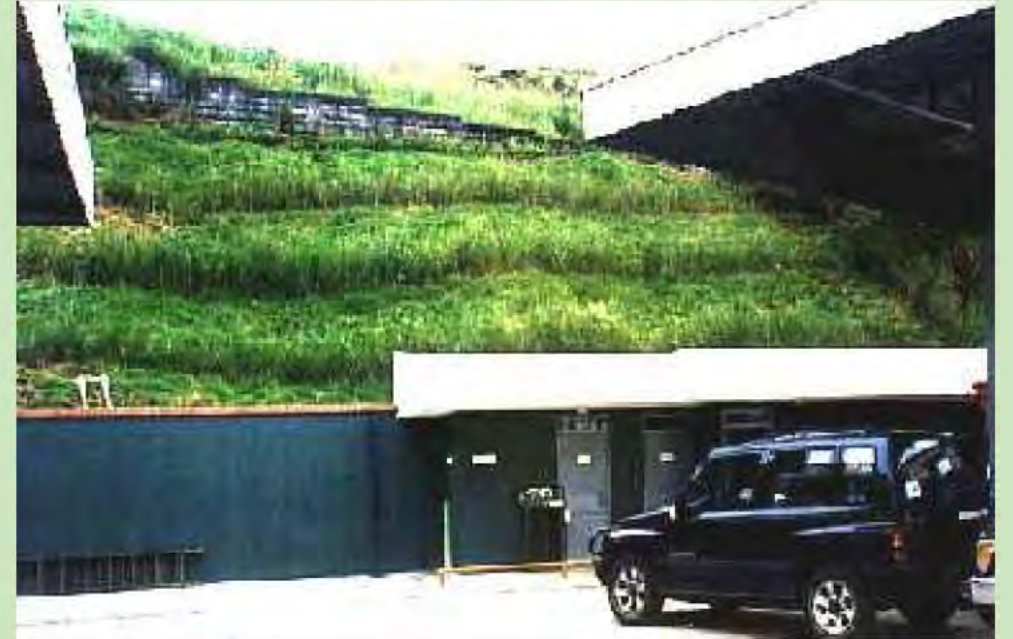
El Salvador - Landscaping and slope stabilization at an urban gas station.
