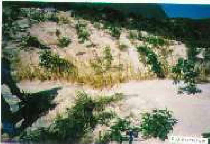
Hong Kong - Kowloon. Above, vetiver hedgerows and Gmelina trees planted on heavily eroded granite surface on fill behind airport. Below, 1994, one year after treatment. Photo credit: R. R. Bruns
