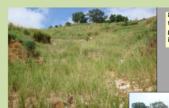
80,000 Sand Bags were used for the stabilisation of the erosion gullies. Vetiver grass was planted into the Sand Bags.
