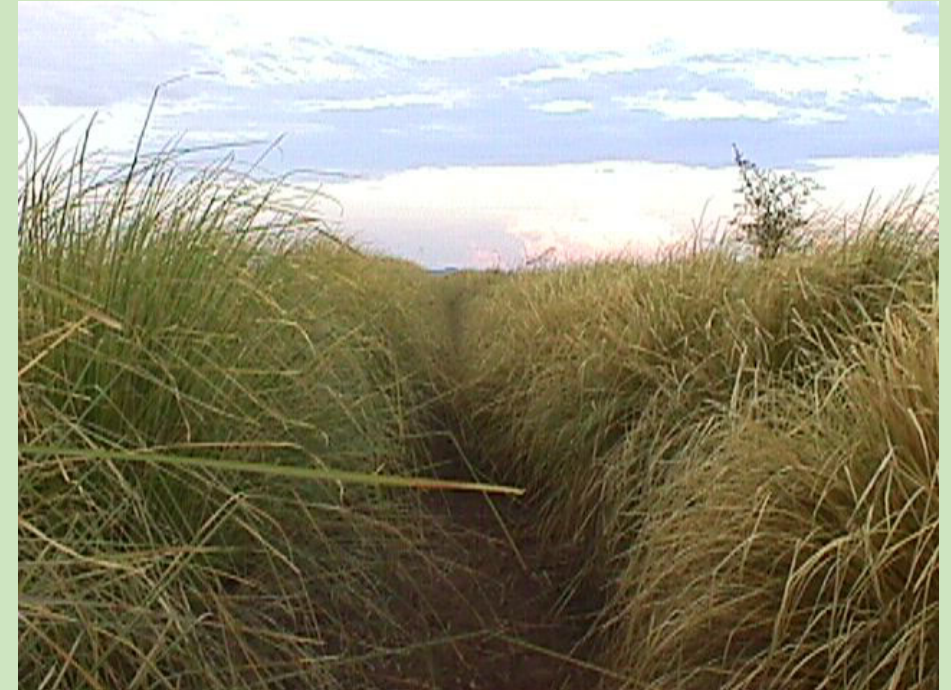
Madagascar - Vetiver stabilizing irrigation canal
