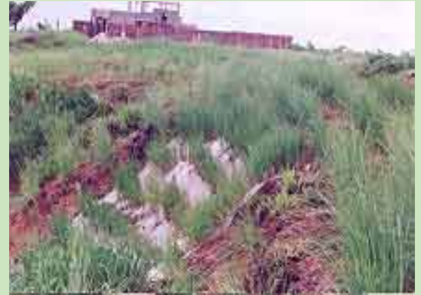
Mexico - Oaxaca. Stabilizing a cliff with vetiver
