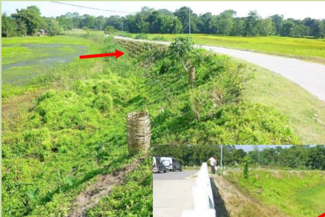
Doria Bridge approach, three years after planting (2011 )
