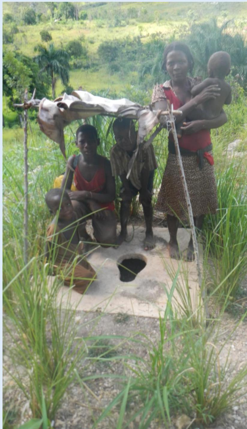
**A Vetiver toilet is simply Vetiver grass slips planted around a small concrete slab above the pit. Instead of bricks and mortar the long roots of the grass stabilize the pit and even remove environmental contaminates.**
