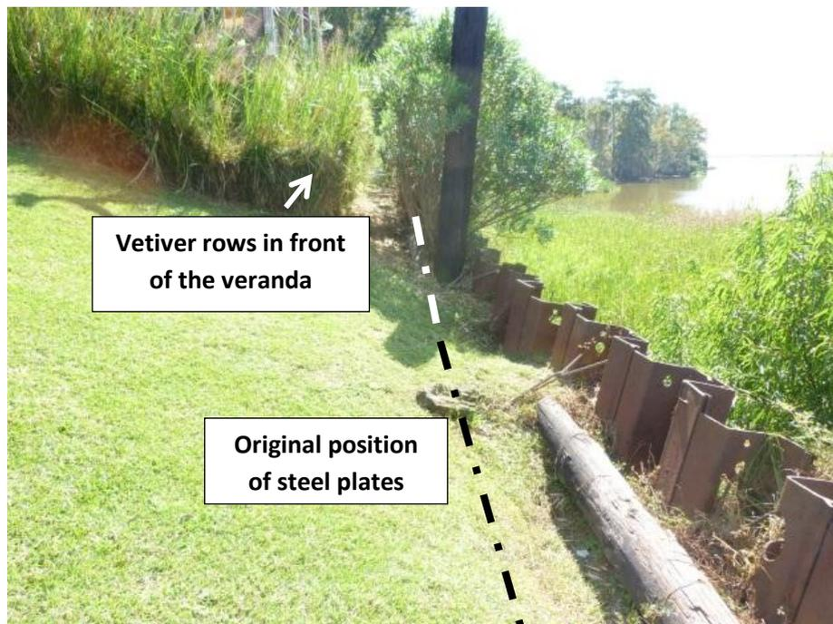
Similarly, on the other side of the restaurant, instead of planting a few rows of vetiver on the affected area, the owner installed anchors to hold up the steel wall to preserve the scenic ocean view.
