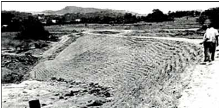
Photo 38b. Vetiver grass planted on this dam wall protects the down slope from erosion.
