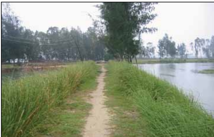
Photo 36. Vetiver hedgerows used to protect both sides of a canal bank in Vietnam. (Tran Tan Van).
