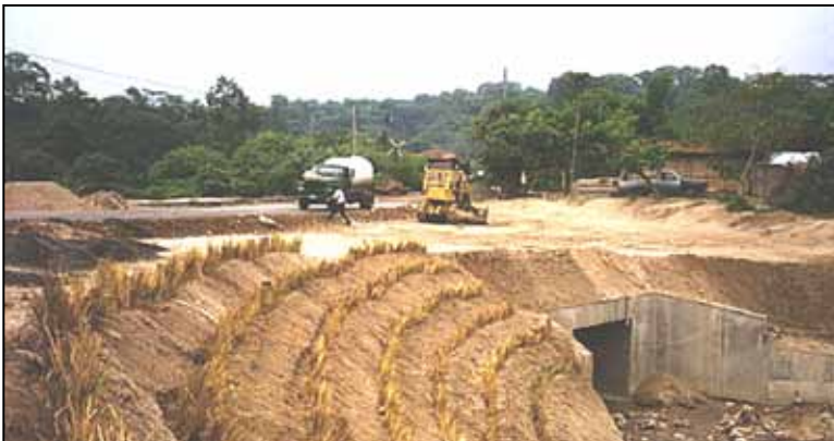
Photo 35. In El Salvador, newly planted vetiver hedgerows protect the approaches to a small bridge.
