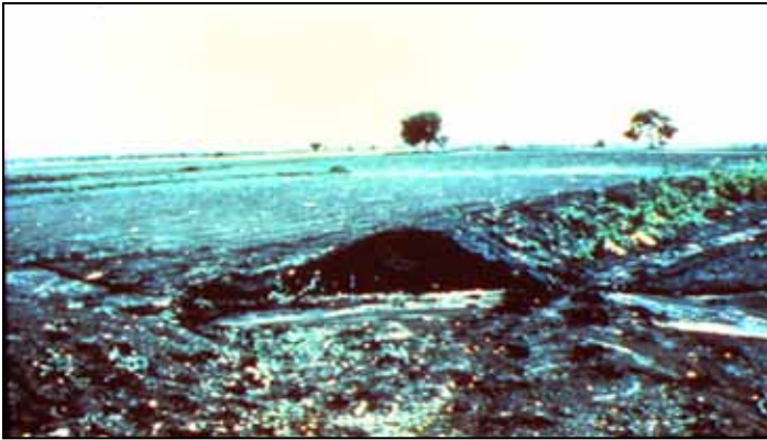
Photo 9a Not only has the constructed bank failed, but the cotton crop that the bank was constructed to protect has also failed. Before this bank's failure, the constructed system trapped too much water, flooding the entire area. Because cotton cannot tolerate poor drainage, the crop failed completely.
