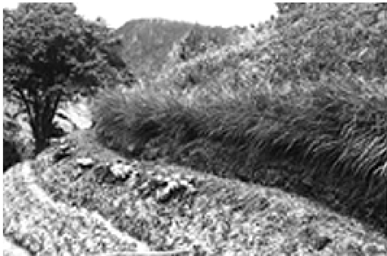
Photo #13: Panama, Cerro Punta. This hedge was established on 100% slope to stabilize farm land in an area adjacent to the Amisconde National Forest. The system works and the farmer is happy with the results. Note how crops are now cultivated on the contour.
