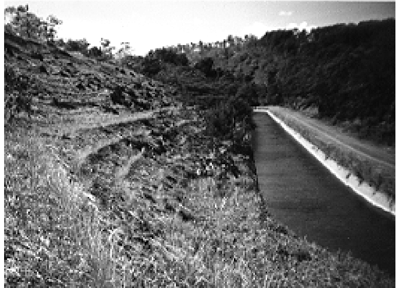
Photo 6: Newly planted vetiver on cut section above canal in Mindanao, The Philippines, used for bank stabilization and control of debris.
