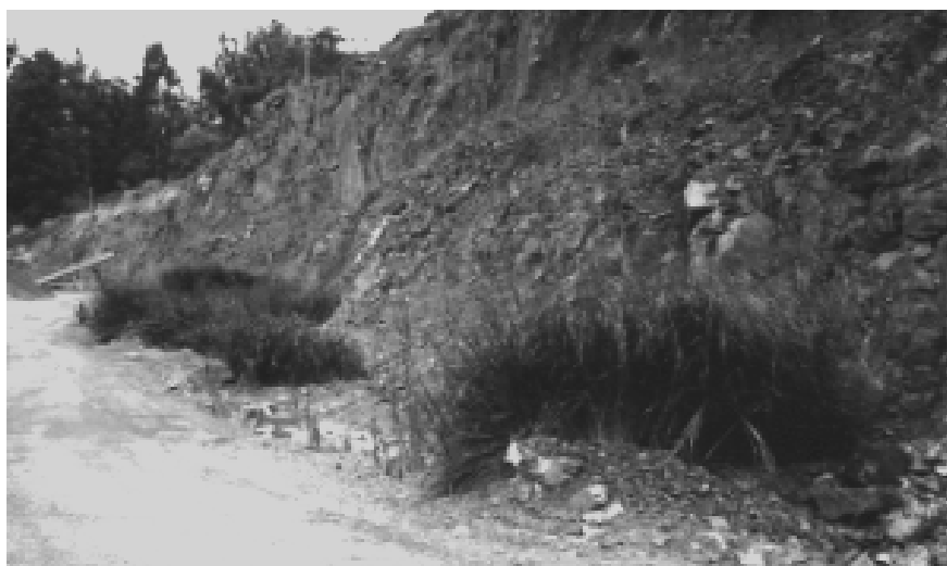
Photo 10: Filter strips in a quarry in Queensland, Australia, filtering sediment from water being discharged into a dam.
