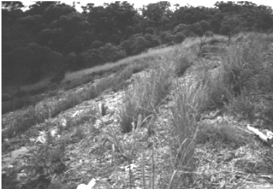
Photo 11: Queensland, Australia. Rehabilitation of toxic municipal waste dump using vetiver grass.
