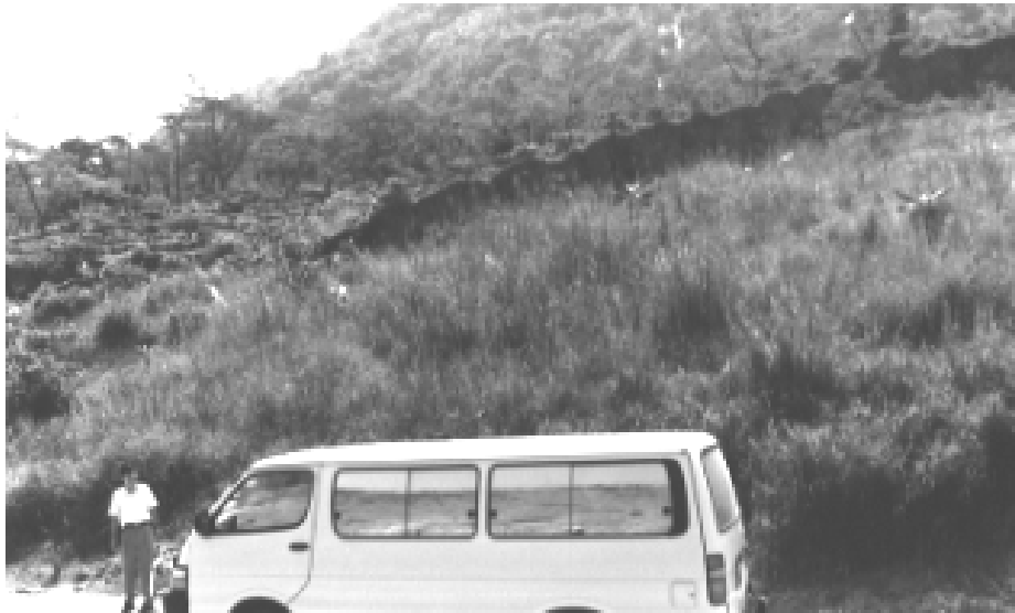
Photo 3: China. Guangdong Province. A slipping highway cut fully stabilized 6 months after planting vetiver grass
