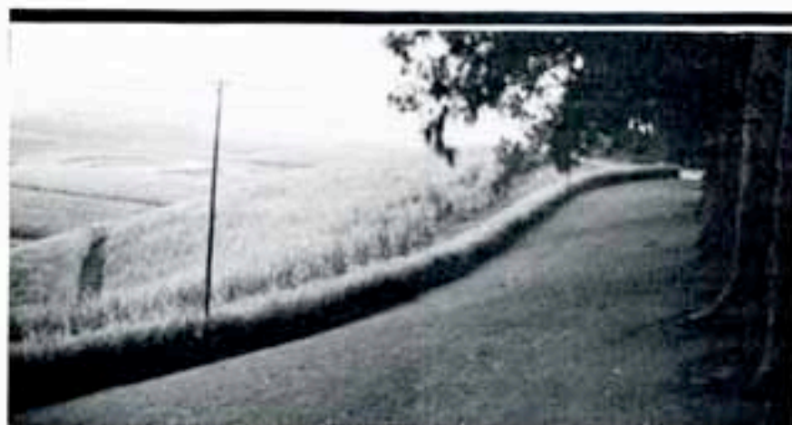
A well established and maintained vetiver hedge planted to control sediment and runoff from a dirt road in Africa.
