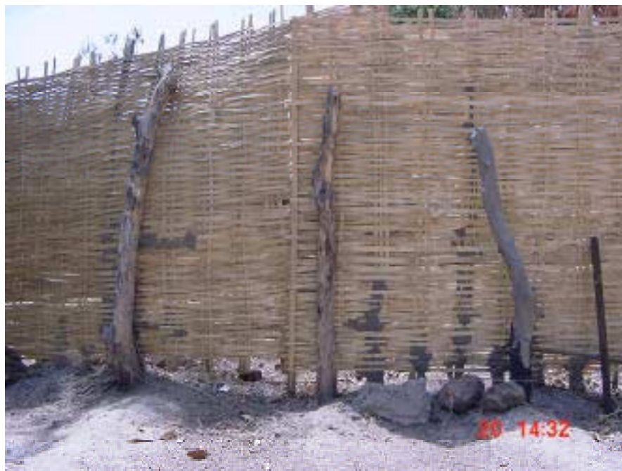
Senegal: v. nigritana : The poles and parts of this enclosure are covered with termite plates showing strong presence of destructive termites.
