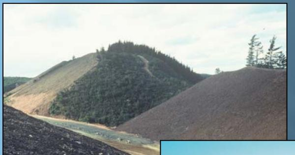
Macchia mulched material placed on side slopes and hydroseeding in progress
