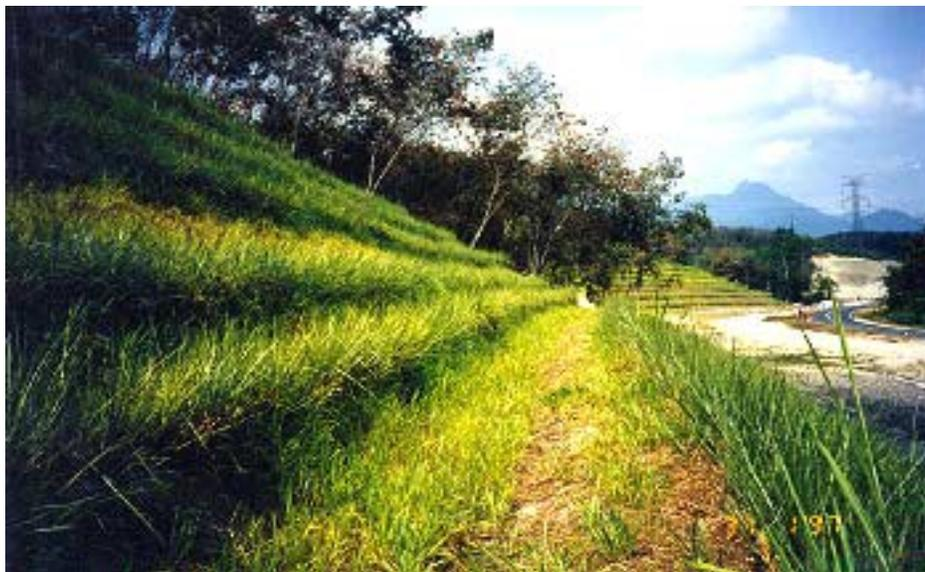
**Figure 16-21. Engineers, who doubted that vetiver roots would penetrate a steep fill, dug and sluiced away the soil on the side of the fill slope to expose the roots. The roots had penetrated to nearly 4 meters through this rough profile and have now stabilized the fill and “nailed” the soil to the slope. The engineers are now satisfied that the Vetiver System works.**
