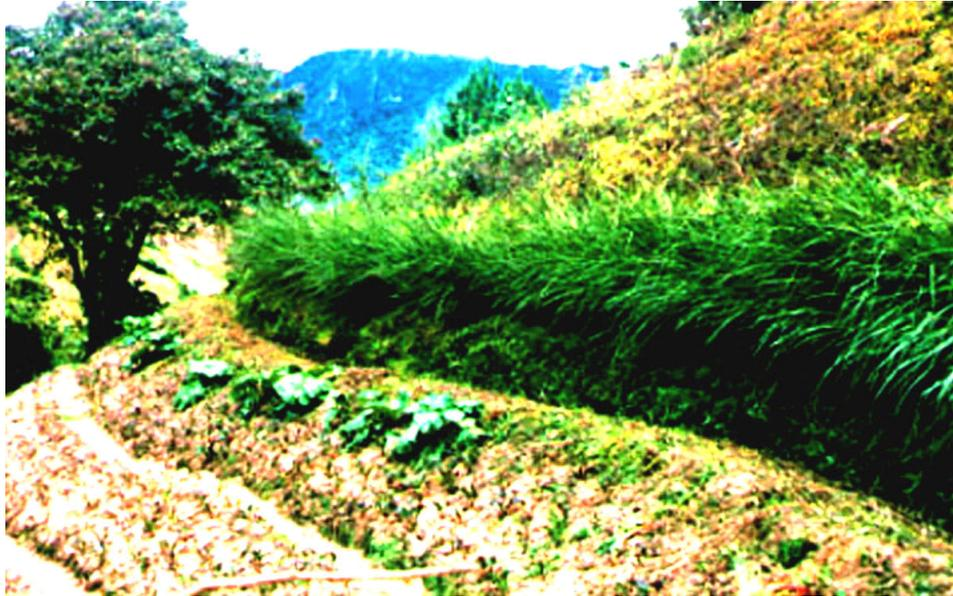
**Figure 16-26. In Natal, South Africa, vetiver hedges, strategically placed down the slope, protect this construction site by preventing rilling from even starting. Over time, native plants will germinate between the hedges, voluntarily stabilizing the whole area, although the vetiver hedges, as they are planted, could do the job alone. The natural regrowth fostered by the hedges prevents wind erosion from blowing noxious dust into the townships.**
