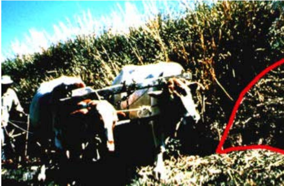
**Figure 16-3b.** This 10-meter-wide constructed soil conservation bank in Maharashtra, India, built just two years earlier on the black cotton soils, has burst. The field officer is standing on the break. The bank cost a lot of money to build, will cost more money to repair, and occupies too much land. It is useless.
