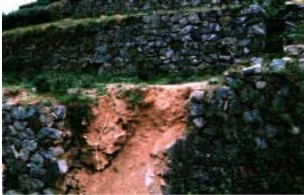
**Figure 7-31b.** A terrace system in the hills can easily be washed out during the rainy season.
