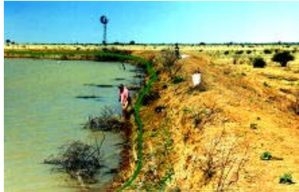
**Figure 16-23b.** At the same Queensland site (as in Figure 16-23a), the vetiver hedge grows despite dry weather, protecting the dam from erosion and preventing silt from entering the dam.
