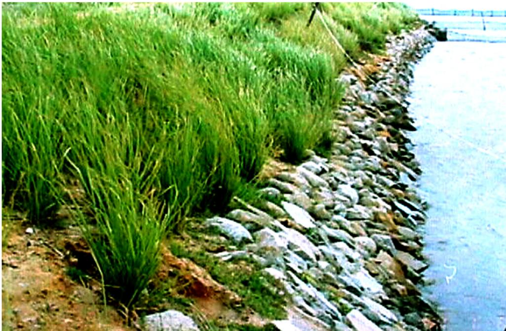
**Figure 16-25. In Panama, a vetiver hedge protects a farmer's vegetable garden from the damage of intense runoff above his field. The hedge will slow down the runoff, spread it out, and prevent it from concentrating in any area, thus preventing erosion, or worse still, slipping.**
