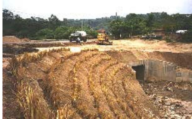
Figure 7-36a shows how vetiver grass can be used to protect the banks of a major irrigation canal. In Bangladesh, as seen in the photo in Figure 7-36b, the canal has been stabilized with vetiver hedgerows for decades, and the plants do not invade the river or the fields behind the rows.
