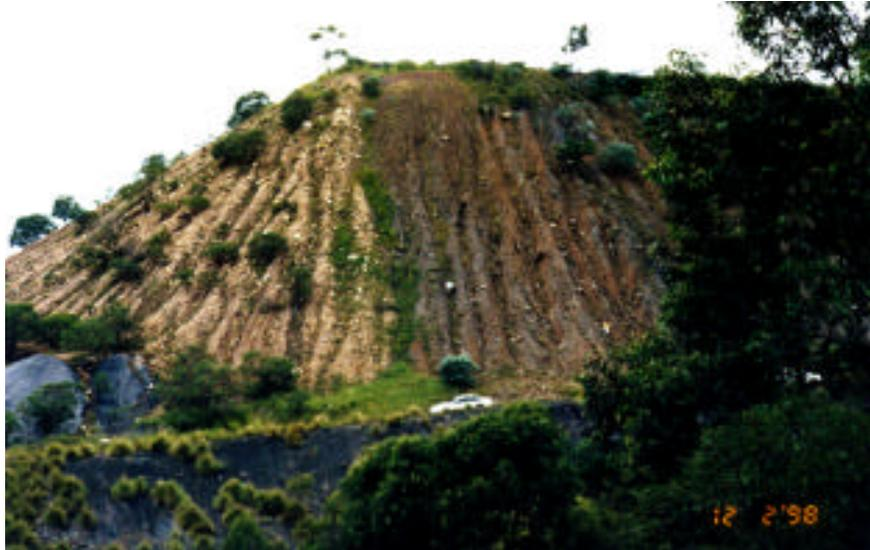
**Figure 16-28b.** At this same site (as in Figure 16-28a), after the Vetiver System was introduced, vetiver plants grow in the larger rills, and hedges thrive on the easier slopes at the bottom of the tailing.
