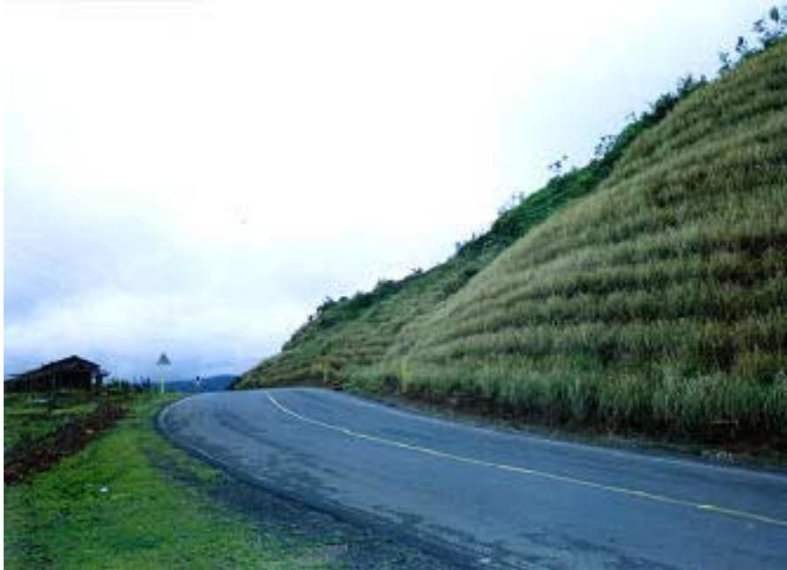
**Figure 16-20b. This road in Malaysia, that suffered severe collapse was eventually stabilized using vetiver hedges, and no further problems have occurred where the hedges were well-established. Nonetheless, engineers were still skeptical, asking for proof.**
