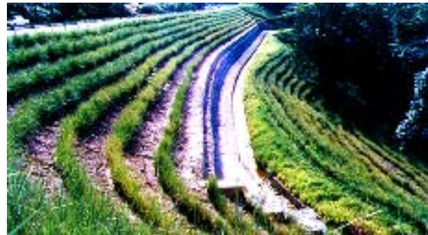
The photos in Figures 7-32b and 7-32c show how vetiver grasses have been used in Malaysia to protect roads. In Figure 7-32b, the hedgerows stabilize the slopes of country roads. Once the hedges are established, the roads are fully stabilized and do not slip. The cost to establish the hedges is minimal, and the maintenance is even less. The same Vetiver System is used to stabilize high-cost highways, as shown in Figure 7-32c.
