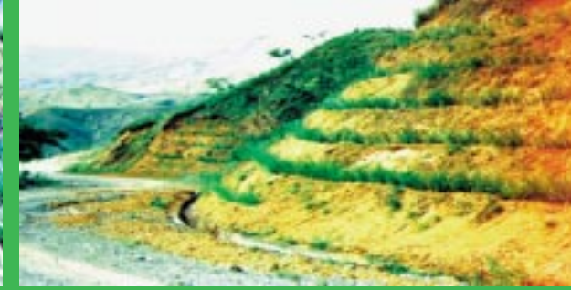
Philippines - VS applied to highway cut that had been seriously damaged by earthquakes
