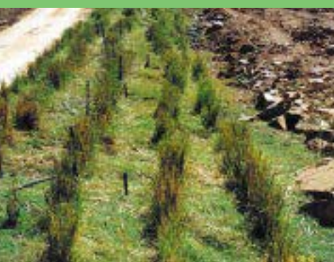
Australia - the same causeway now stabilized with vetiver grass hedgerows. Damage by flooding minimized
