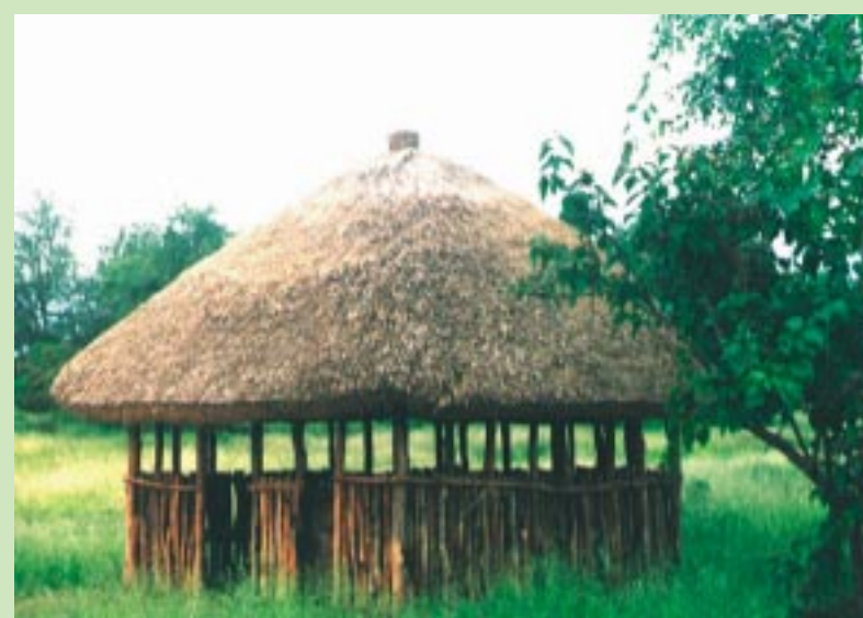
Zimbabwe - a nicely thatched meeting house using vetiver grass thatch. The thatch will last three times as many years due to its resistance to insects and fungus attack
