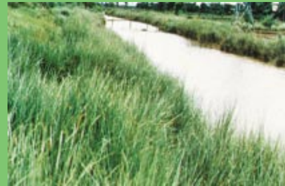
Bangladesh - irrigation canal protected with VS. Vetiver has been here for many years, and has shown no sign of escape
