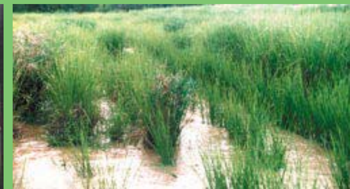
Zimbabwe - vetiver grass hedgerows were planted across a 100 meter wide reservoir spillway. The spillway was subjected to 3 months continuous flow
