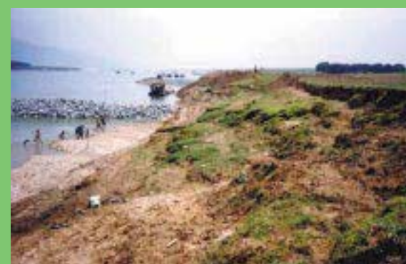
China - river flood embankments become heavily eroded and often breach causing much economic damage
