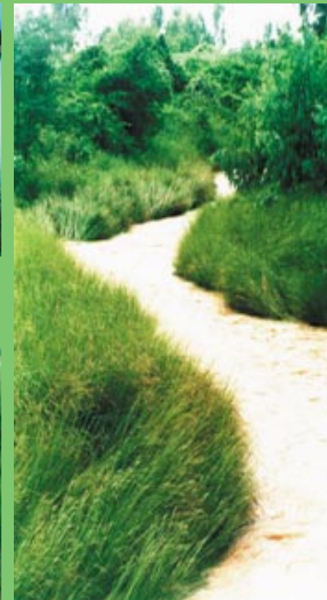
Zimbabwe - a fast flowing stream protected from stream bank erosion using VS application
