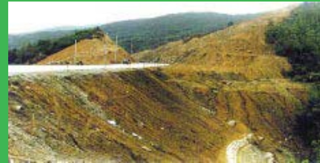
China - unstable highway fill prior to VS treatment. Road stability was so bad in untreated state that major lateral cracks in the pavement occurred
