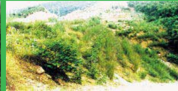
China - same fill less than a year later. After another two years this fill became fully forested. Untreated cut shown as white in background
