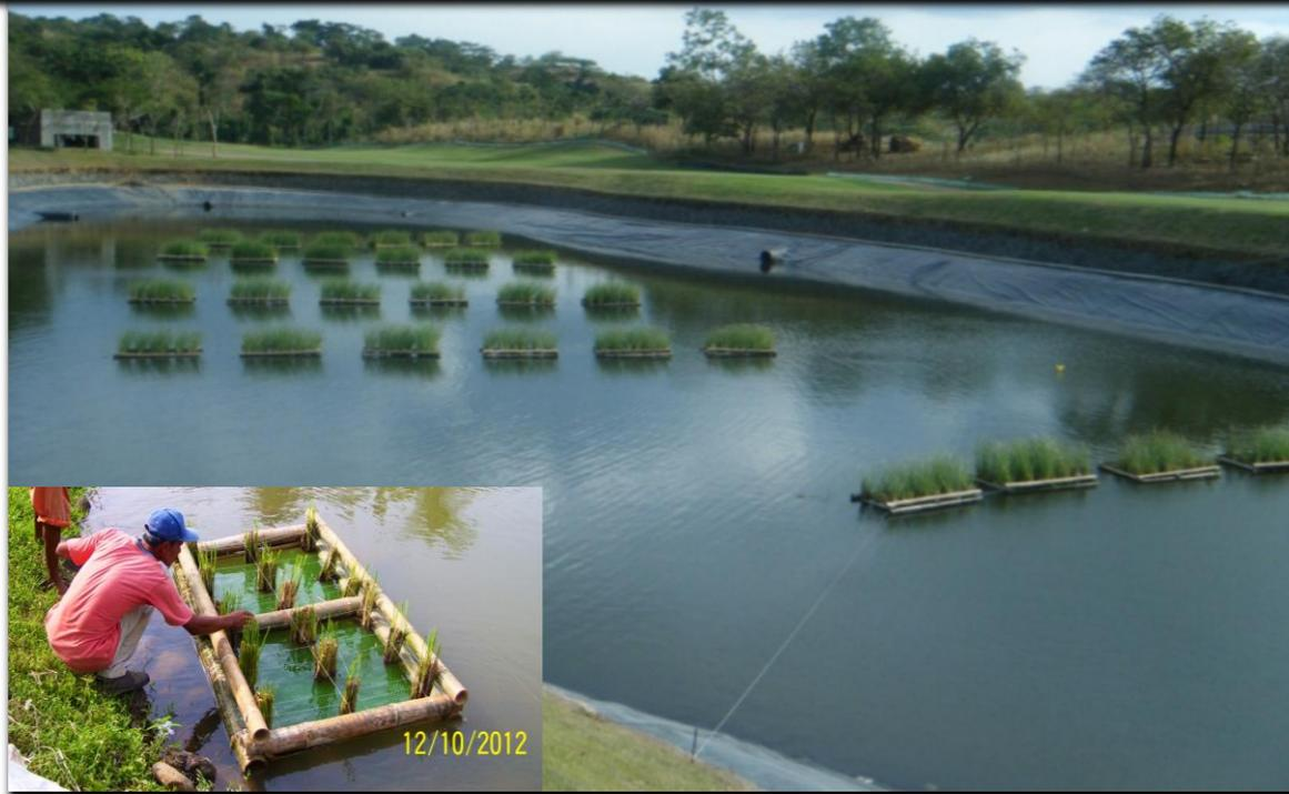
**Bamboo Pontoon (2 x 1 meters) For water treatment**
