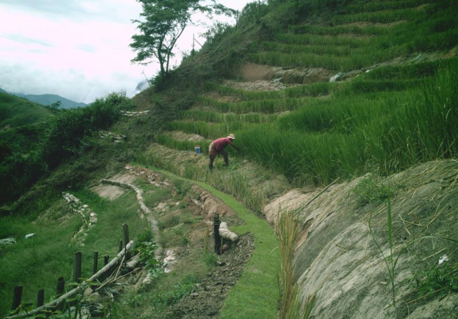
Vetiver planting has successfully stabilized this landslide
