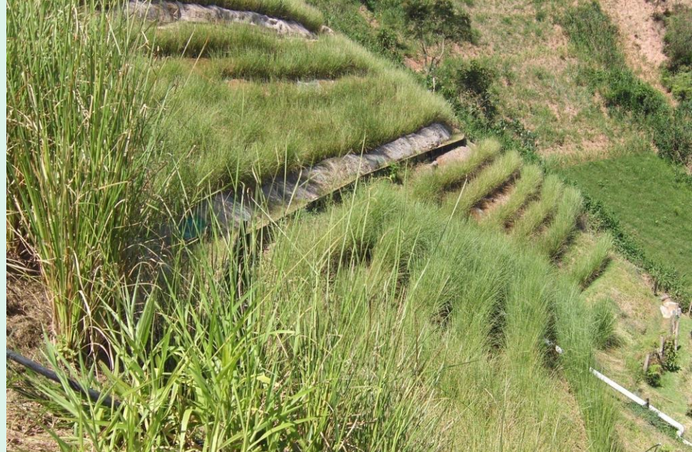
Vetiver planting has successfully stabilized this landslide
