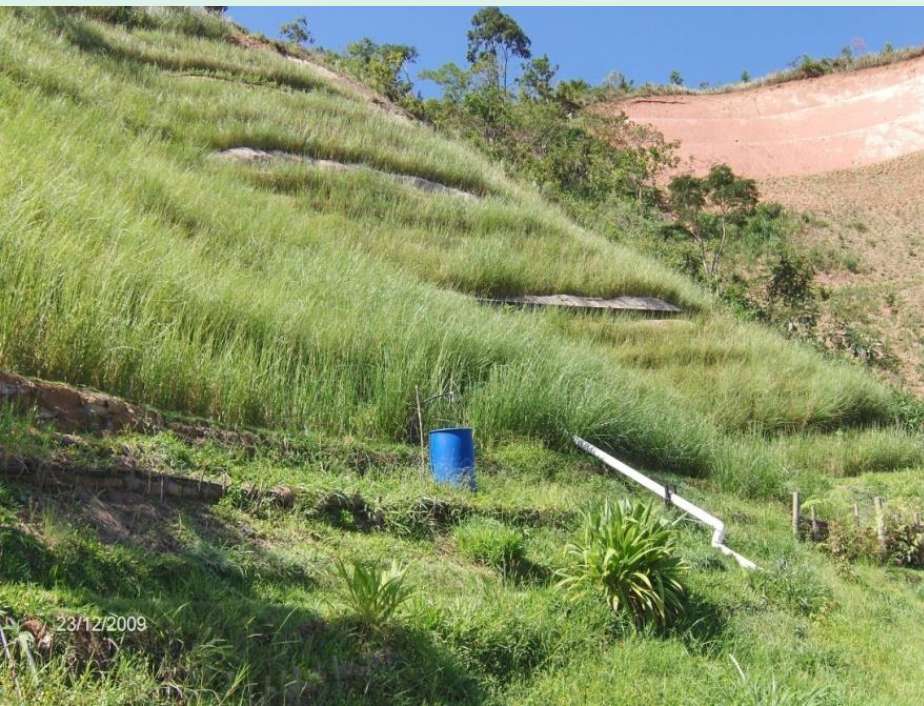
Vetiver planting has successfully stabilized this landslide
