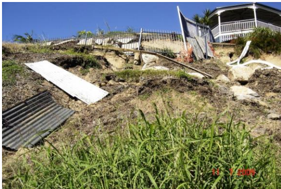
Landslide threatened the foundation of this house on a very steep hill. The slope was repaired and vetiver planting provided full protection two years after planting
