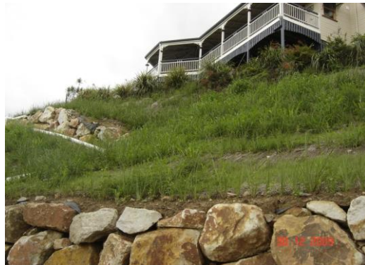
Landslide threatened the foundation of this house on a very steep hill. The slope was repaired and vetiver planting provided full protection two years after planting
