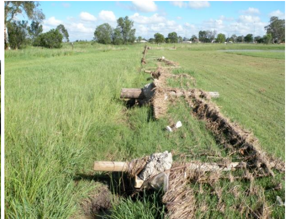
Eight year old Vetiver hedges undamaged and fully protected the drain, while the concrete footed fence was ripped up by the big flood
