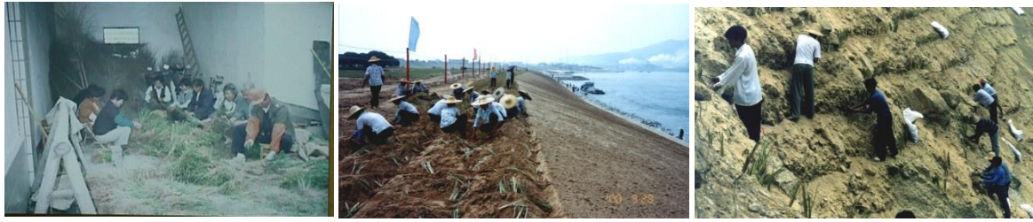
Female local workers preparing vetiver slips and planting on the riverbank and male workers planting on the steep slope
