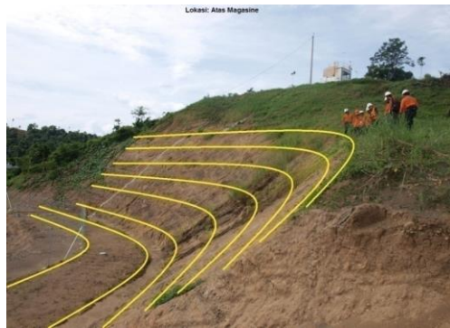
Photo 22: Vetiver application at PT Meares Soputan Mining, Toka Tindung gold mine site
