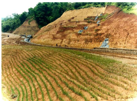
Figure 7: Vetiver were planted as pioneer plant on barren land for highway construction project.
