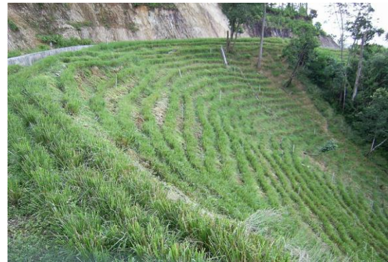
Figure 4: Vetiver planting at the side ditch lining.
