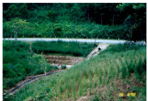
Figure 6 : VS was associated with gabion wall in the rehabilitation work.
