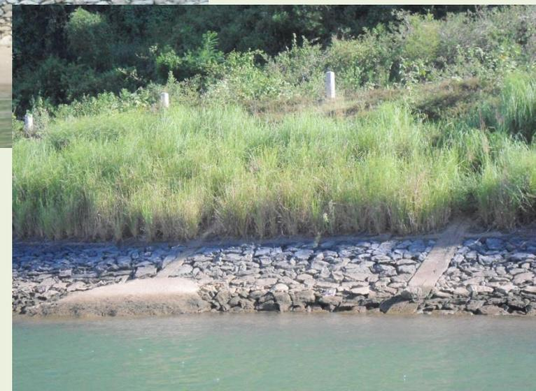
**This is the bank of a coastal river mouth, subjected to full tidal fluctuation. Rock basket was used below high water level and Vetiver planted above to protect the bank from tidal surge during storms and typhoon season.**
