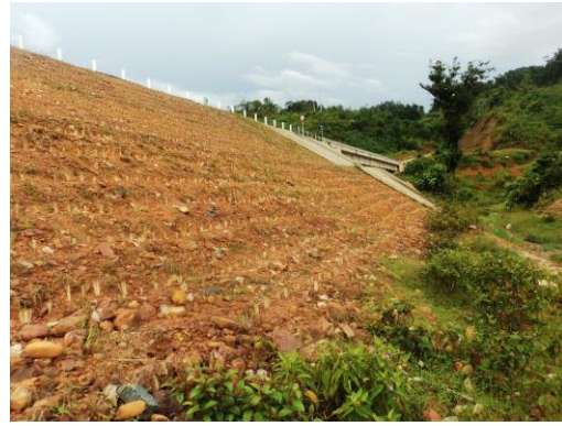
Vetiver planting on contour line on steep road batters
