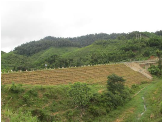
First trimming six months after planting to encourage tiller development
