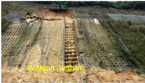
Without vetiver protection the concrete cellular surface protection measure failed
