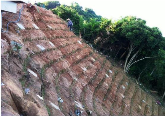
Vetiver planting with soil nailing at Laguna Resort in Huế, before and after
