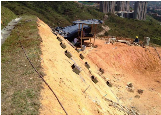
Vetiver planting with soil nailing at Medellín, Colombia , before and after
