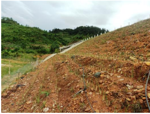
Vetiver planting on contour line on steep road batters
