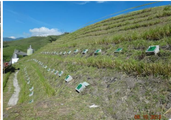
Vetiver planting with soil nailing at Medellín, Colombia , before and after
