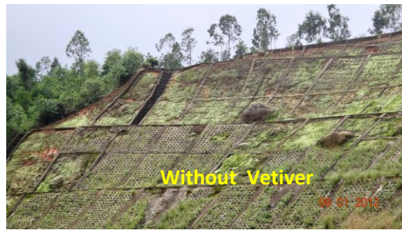
Without vetiver protection the concrete cellular surface protection measure failed
