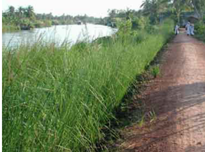
Figure 1.4: Use of Vetiver grass for bank stabilisation
