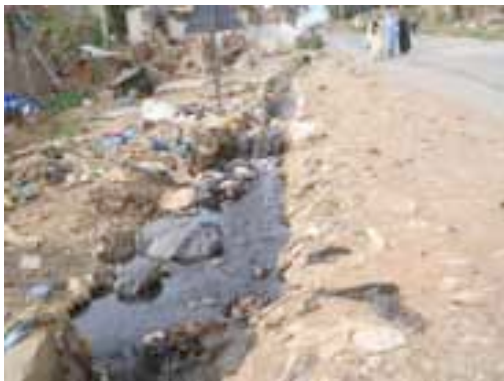
Foul odor leachate stream runs downhill
