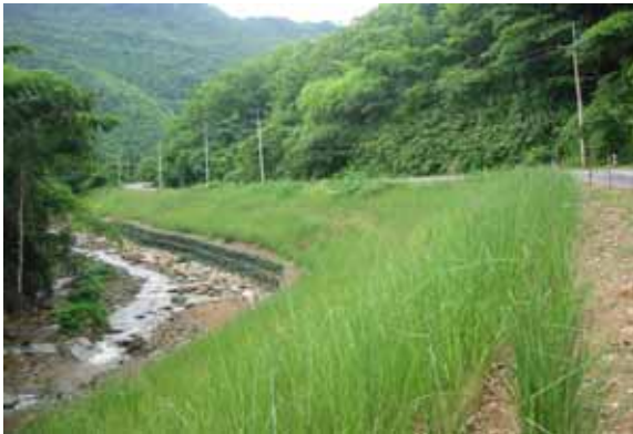
Figure 3 : Stabilization with vetiver along the stream bank.
