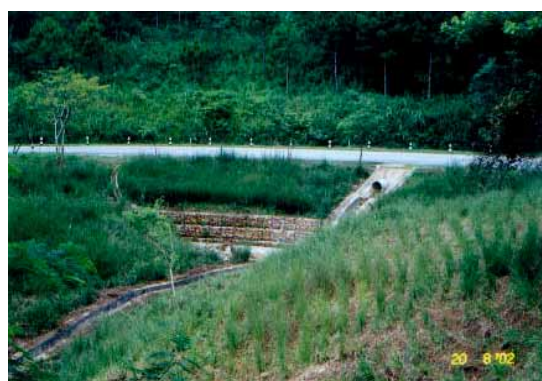
Figure 6 : VS was associated with gabion wall in the rehabilitation work.
