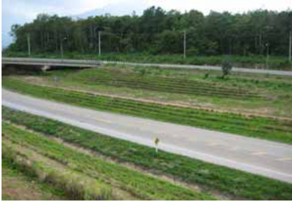
Figure 1: Highway cut slope (back slope) was stabilized with vetiver.
