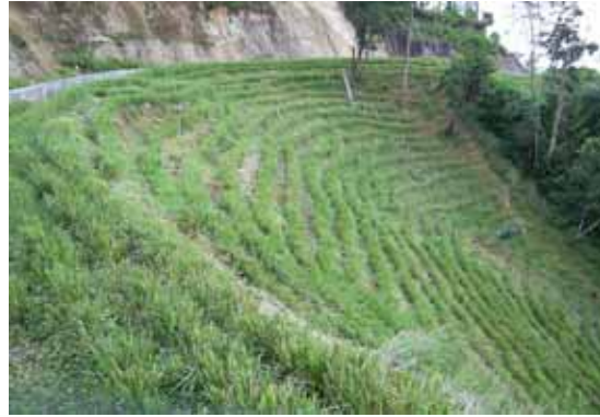
Figure 2 : Highway embankment (side slope) was stabilized with vetiver.
