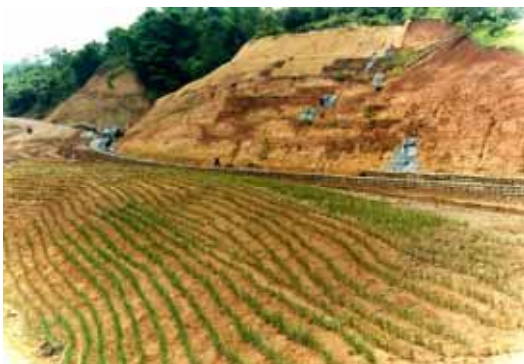
Figure 7: Vetiver were planted as pioneer plant on barren land for highway construction project.
