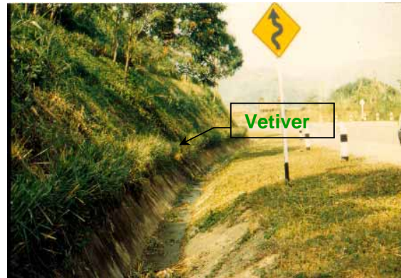
Figure 4: Vetiver planting at the side ditch lining.
