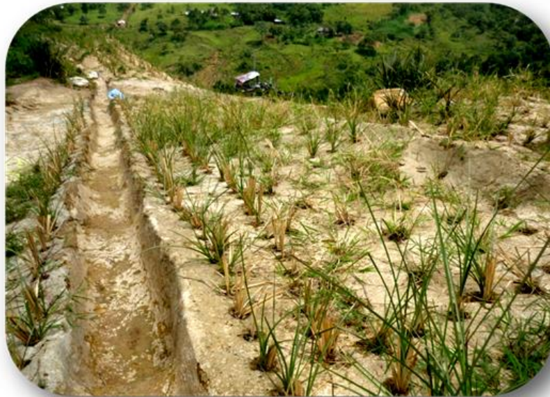
Vetiver. Carretera: Angelópolis – Amagá K 4+100 “Curva del Chocho”
