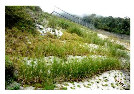
With these good results, the perfect interaction between Vetiver and the Eco Mortar was demonstrated in different soil conditions. The Eco mortar working on the steep slopes of hillside controlling surface erosion and water infiltrations and Vetiver System working from inside the soil giving strength and binding soils. More than  $50.000 \text{ m}^2$  of eroded area has been recovered in a wide range of climatic conditions and different altitudes from sea levels to 2,800 m above sea level
