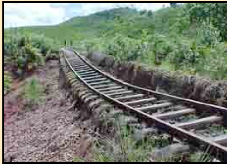
Typical damage from cyclones
