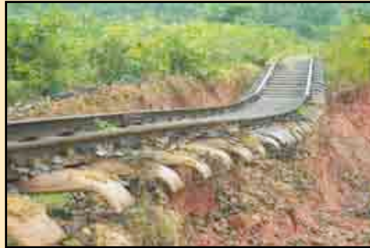
Typical damage from cyclones
